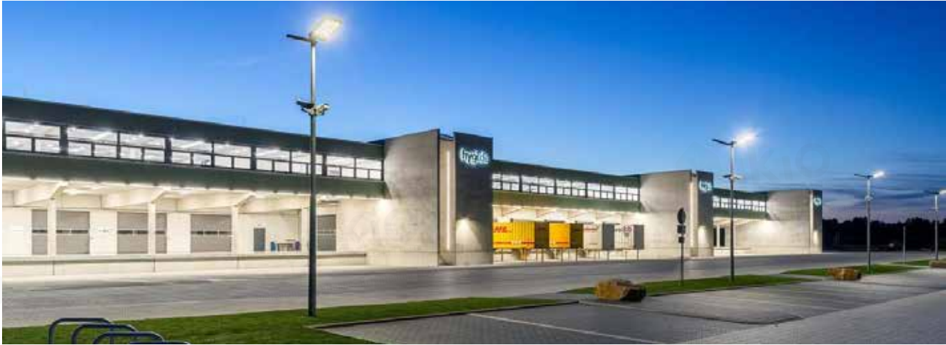
Figure 57. Area Luminaires in a parking lot
