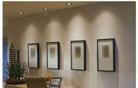
Figure 141. Accent lighting focussed on paintings
