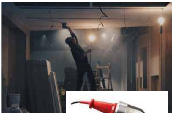
Figure 73. Work lights in use at a construction site
