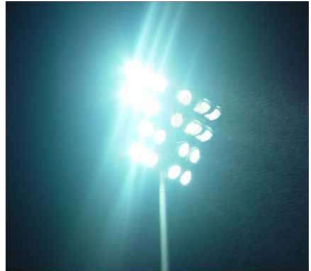
Figure 134. Glare from sports lighting in a stadium
