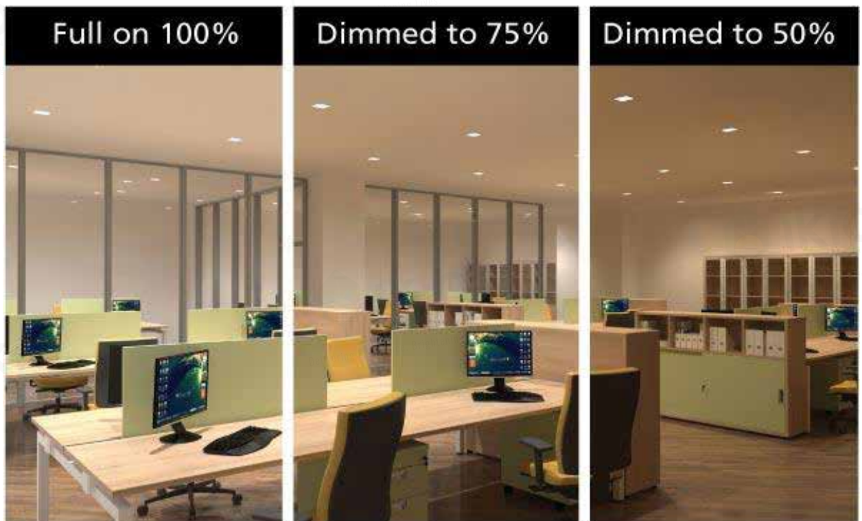
Figure 32. Effects of dimming LED downlights at various levels
