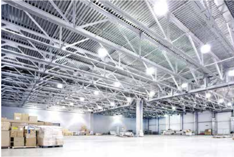
Figure 51. High bay lighting in a warehouse
