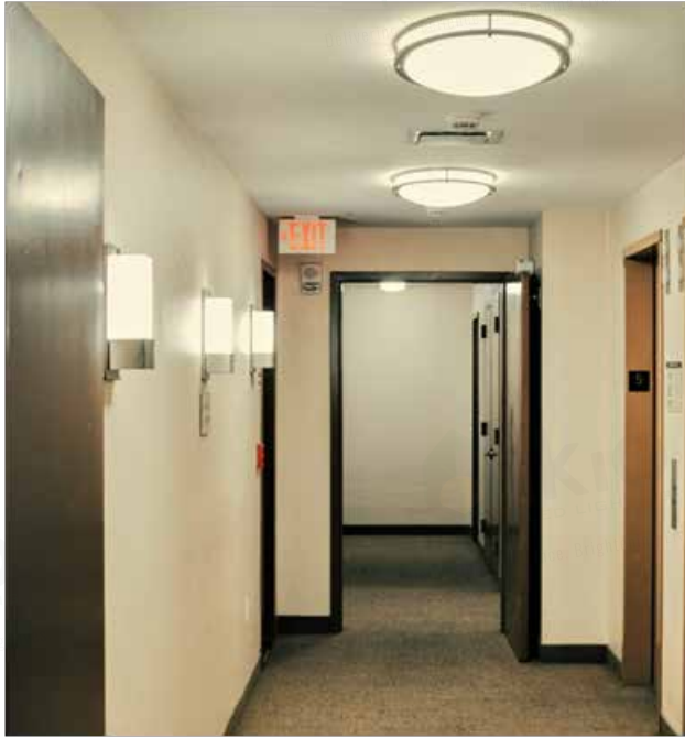
Figure 94. A hallway with flush mount lighting and sconce lighting
